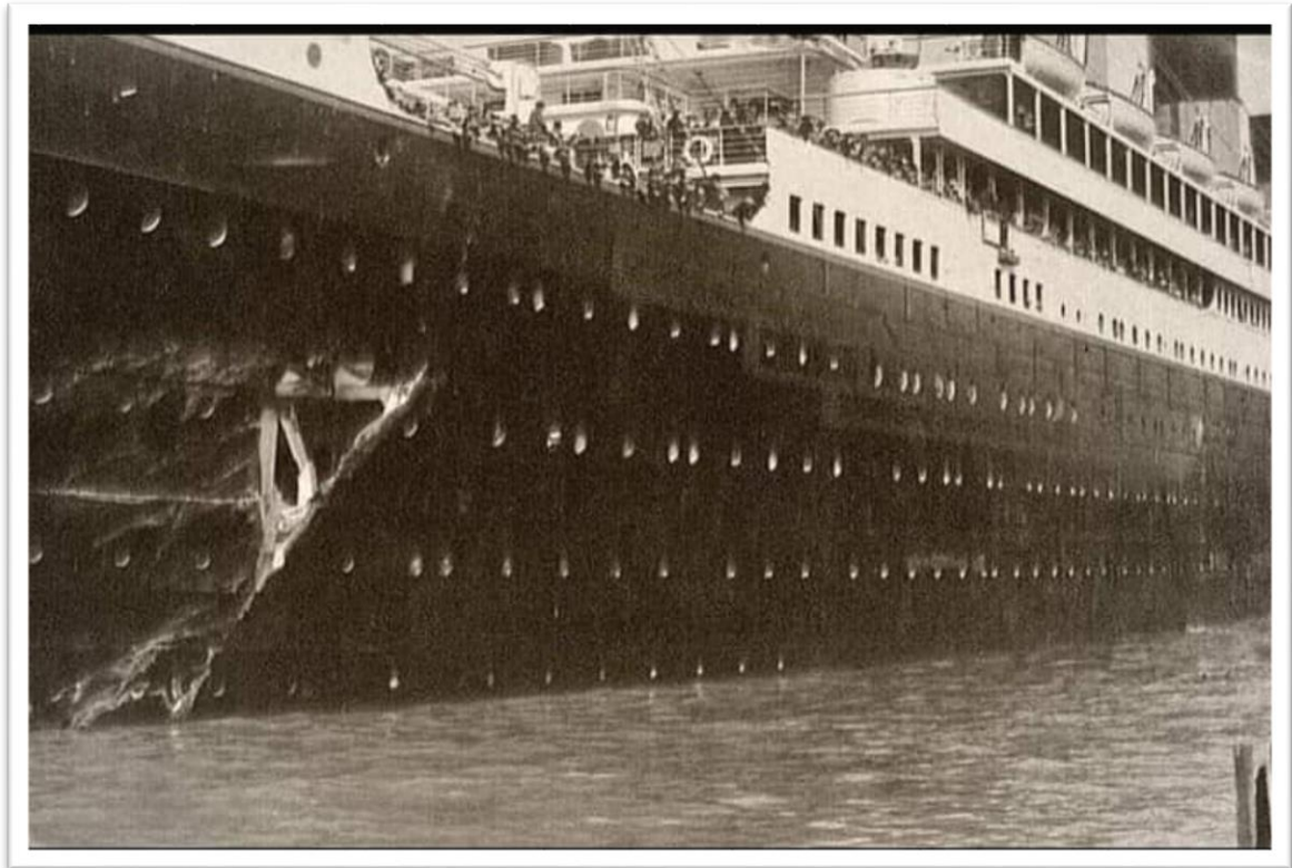
Figure 4: Olympic after her collision with the H. M. S. Hawke. Photo: Public domain image.
